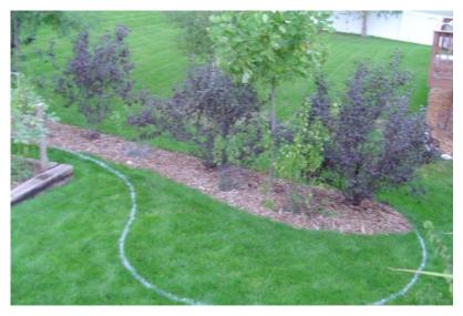
paint or flags. Remember, the size was determined using an average 1 inch storm so if you need to make it slightly bigger or smaller, that's fine. It will either hold a little more or a little less runoff. The garden will have an inflow area where runoff will enter and an outflow area in case you receive more rain than the garden is designed for. Identify these 2 spots when laying out your rain garden. This is where you will incorporate some rocks.
