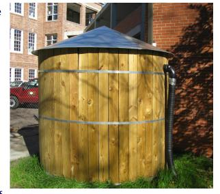
A quick calculation for determining how many gallons of water runs off your roof from a 1 inch storm is  $V = A \times 0.6$ . Volume = gallons of
