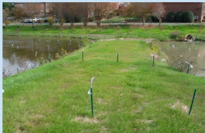
Figure 3. A wide path is provided for heavy equipment to access the forebay (located to the right of the path).
