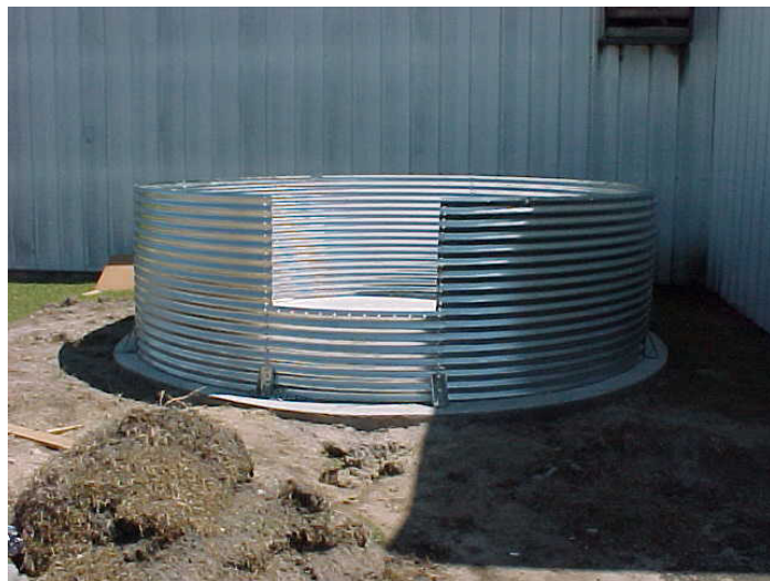
Figure 2. Metal rainwater cistern being assembled
