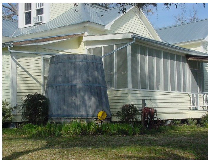
Figure 5. Above-ground cistern located at the corner of a house near existing downspouts (image courtesy of LSU Ag Center)
